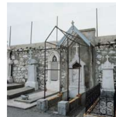
Wrought Iron House , Ancey, France
